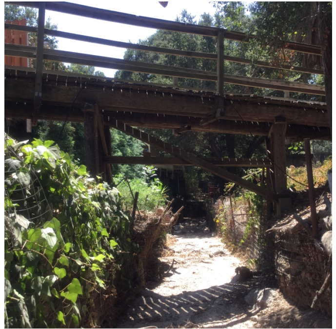
Looking downstream at Str. 14
