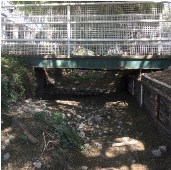
Looking upstream at Str. 2
