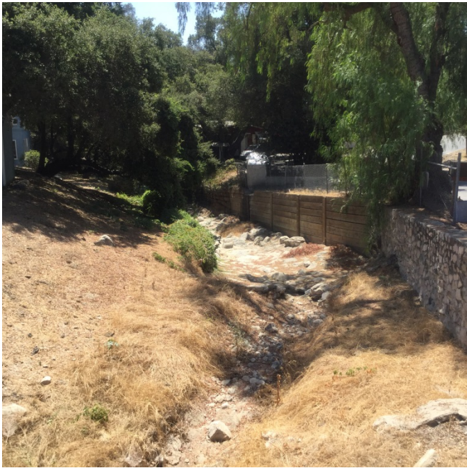
Looking downstream at Kagel Canyon channel from Str. 6 (East Trl)
