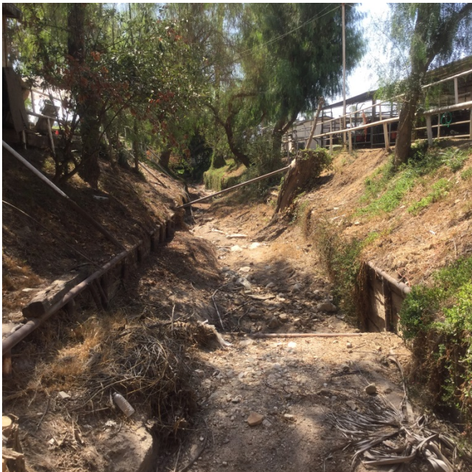
Looking downstream at Kagel Canyon channel from Str. 3
