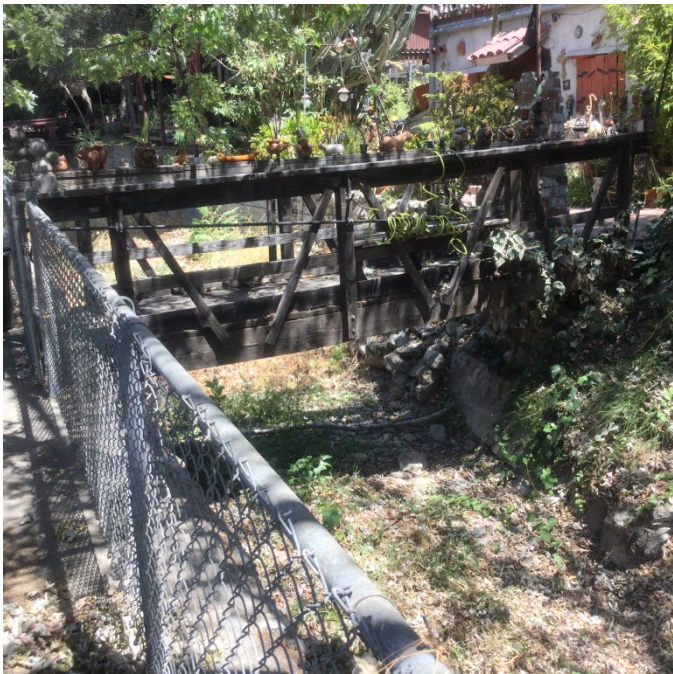
Looking upstream at Str. 9
