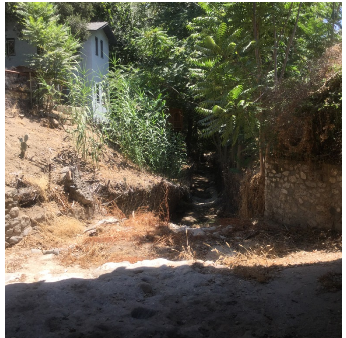
Looking downstream at Kagel Canyon channel from Str. 13
