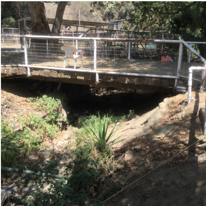
Looking upstream at Str. 4
