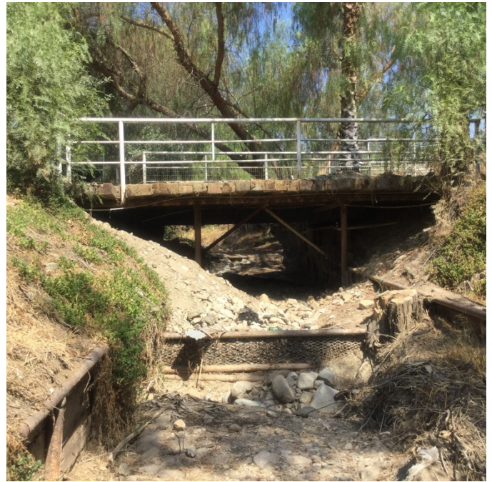
Looking upstream at Str. 3
