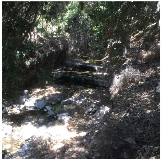
Looking upstream at Kagel Canyon channel from Str. 12
