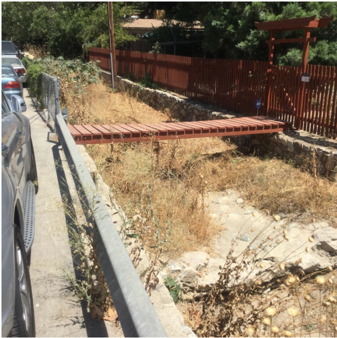
Looking upstream at Str. 7
