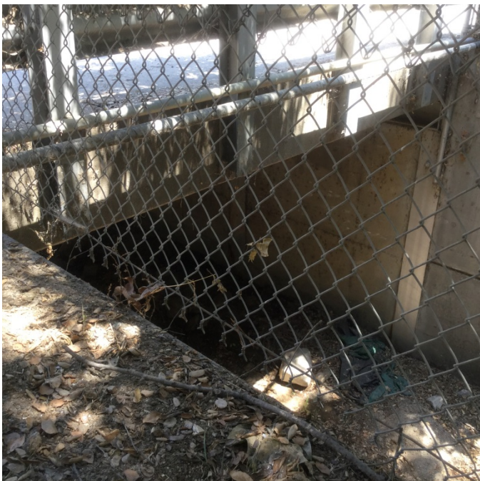
Looking upstream at Str. 12
