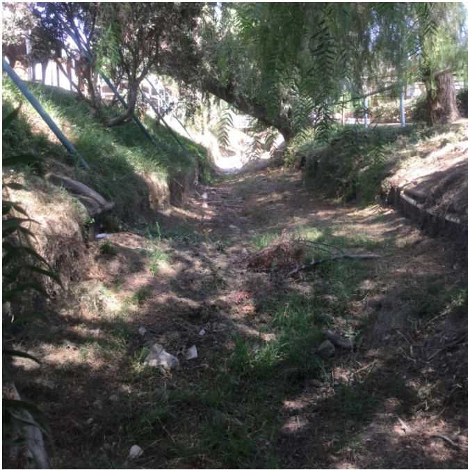
Looking upstream at Kagel Canyon channel from Str. 2
