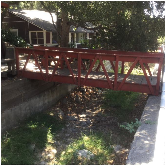
Looking downstream at Str. 10.5
