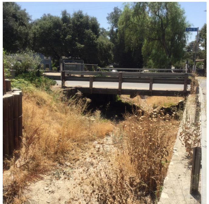
Looking downstream at Str. 6 (East Trl)
