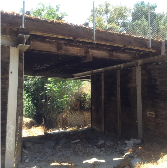
Looking upstream at Str. 13
