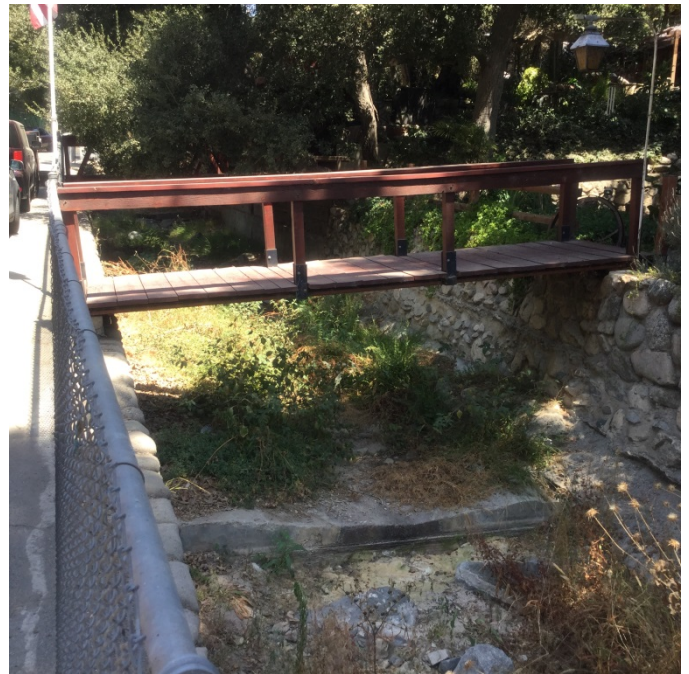
Looking upstream at Str. 10
