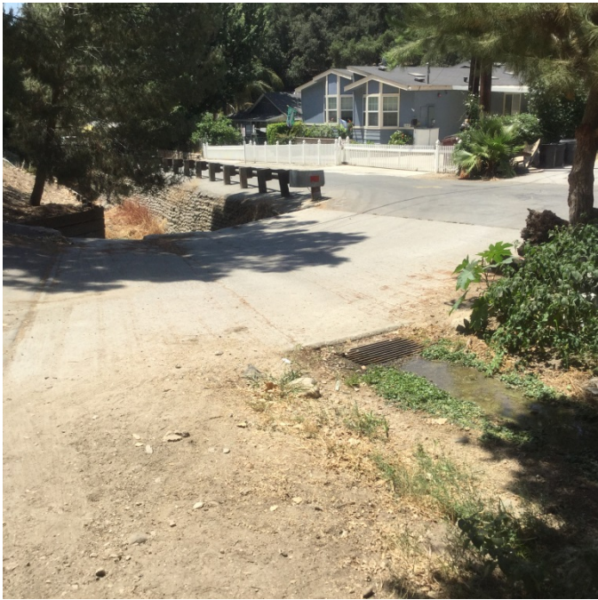
Looking downstream at Str. 11 (Orchard Trl, low water crossing)
