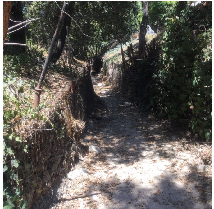
Looking upstream at Kagel Canyon channel from Str. 14
