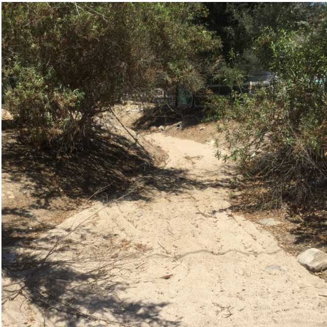
Looking upstream at Kagel Canyon channel from Str. 15 (Blue Sage Dr)
