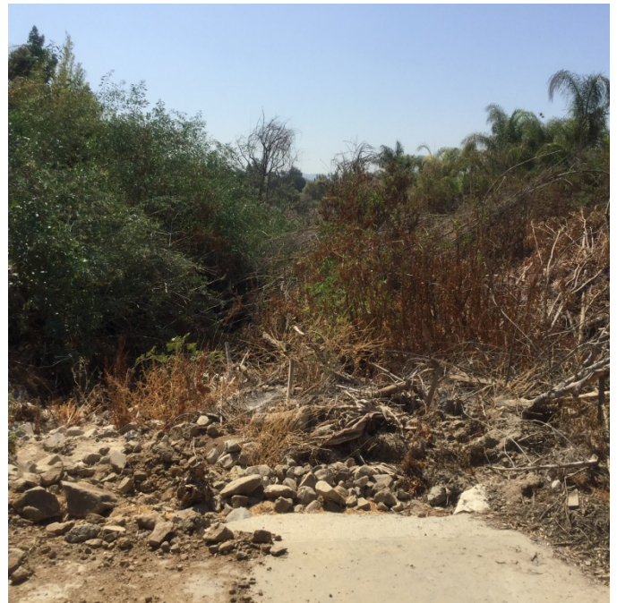
Looking downstream at Kagel Canyon channel from Str. 1 (Osborne St.)
