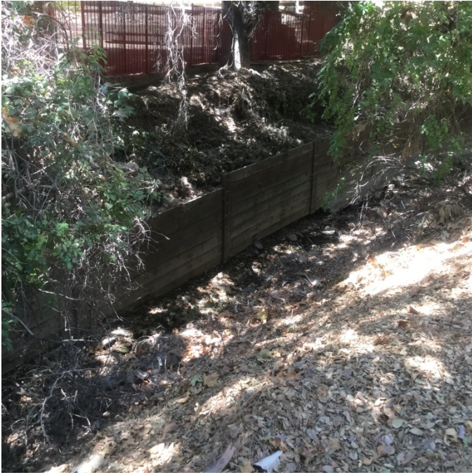
Looking upstream at Kagel Canyon channel between Str. 12 and 13
