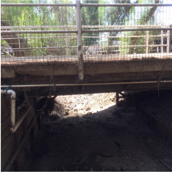
Looking downstream at Str. 3
