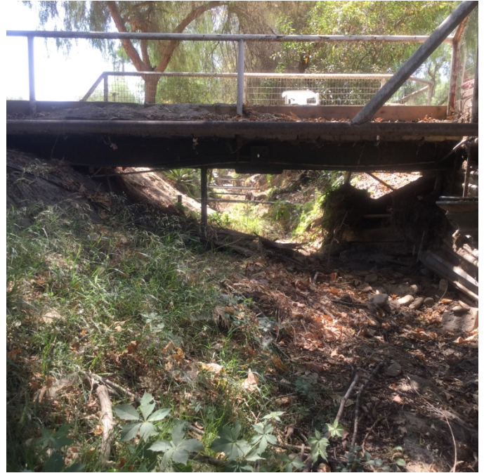
Looking downstream at Str. 4
