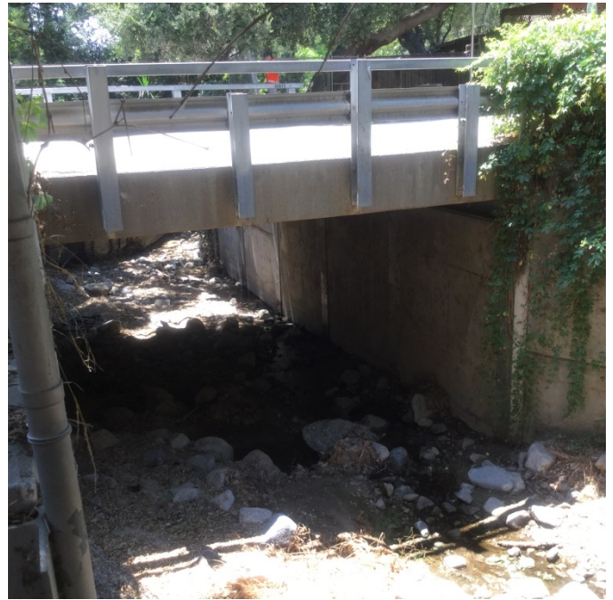
Looking downstream at Str. 12
