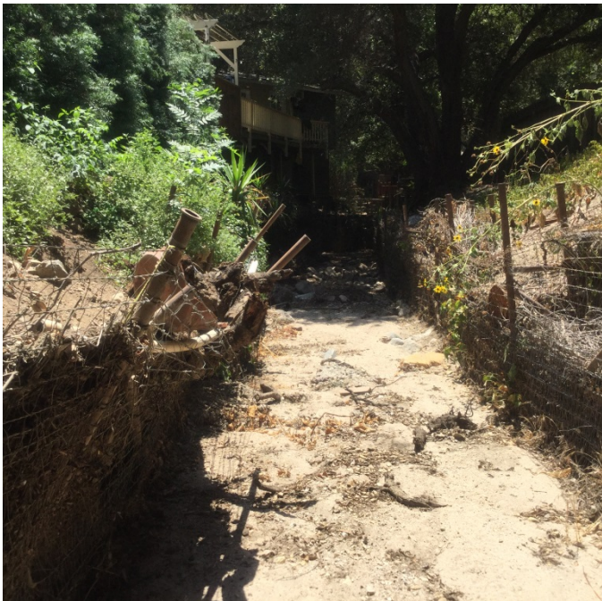
Looking downstream at Kagel Canyon channel from Str. 14
