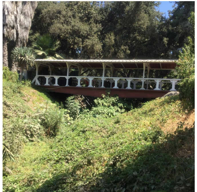
Looking upstream at Str. 5
