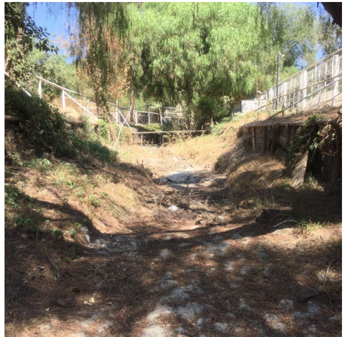
Looking upstream at Kagel Canyon channel from Str. 3
