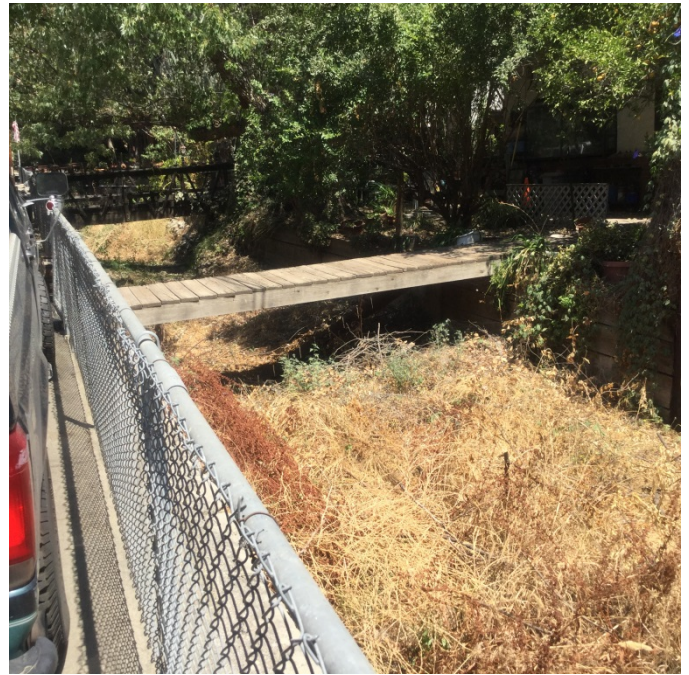
Looking upstream at Str. 8
