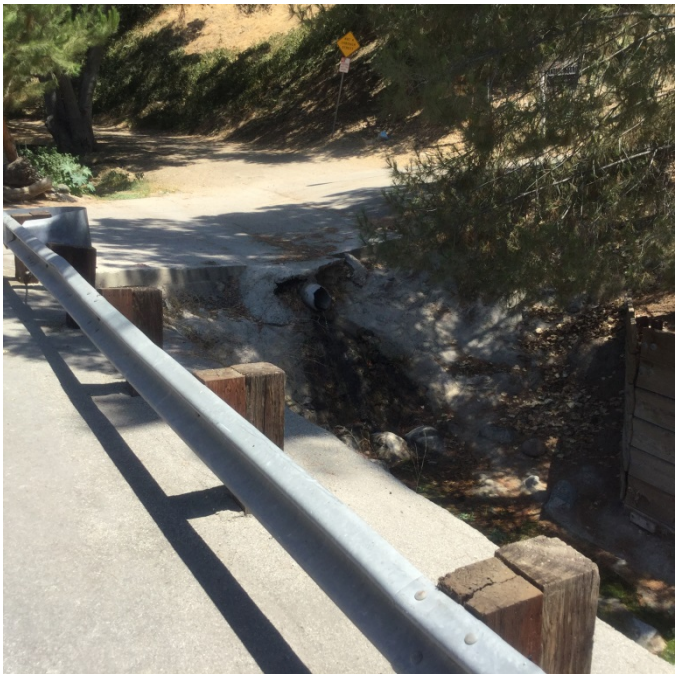
Looking upstream at Str. 11 (Orchard Trl, low water crossing)
