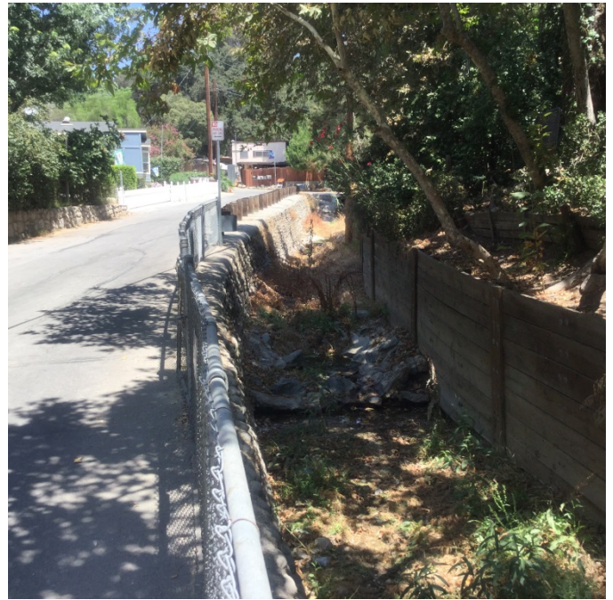
Looking upstream at Kagel Canyon channel from Str. 10.5
