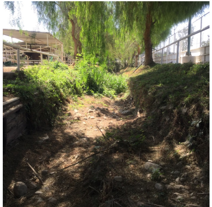
Looking downstream at Kagel Canyon channel from Str. 2
