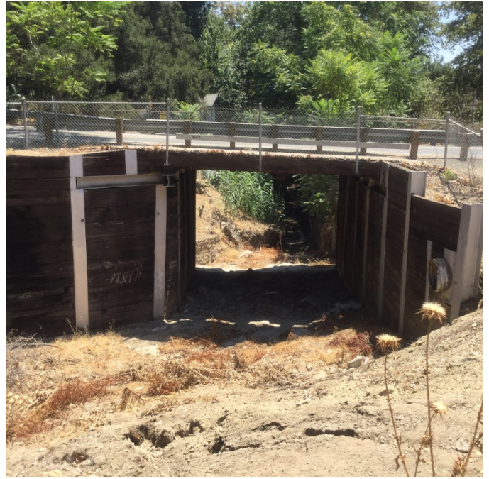
Looking downstream at Str. 13
