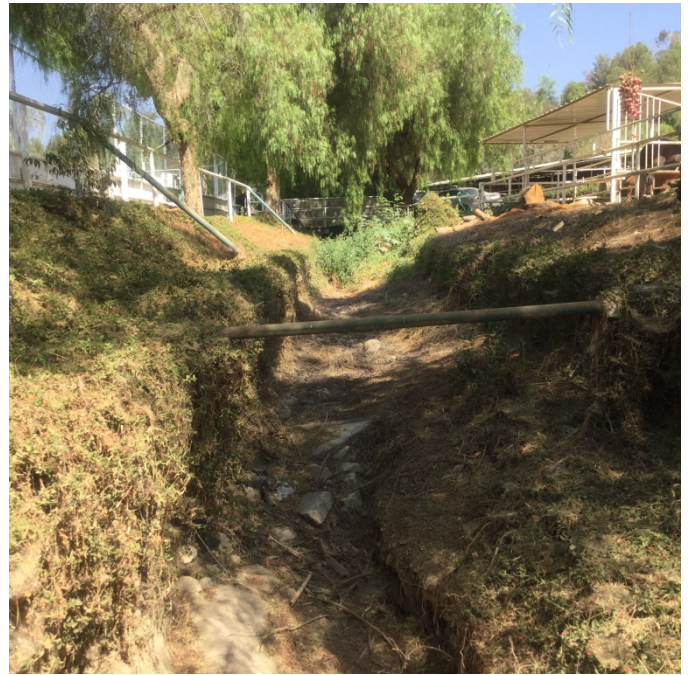
Looking upstream at Kagel Canyon channel between Str. 1 and 2
